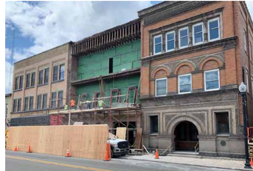
The existing building, pictured in the middle, had been vacant since 2015.
