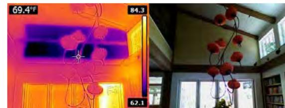
Poe Street Passive House, Paolo Alto CA. One and a half Ray Magic panels installed on the wall seen through infrared camera in cooling.
