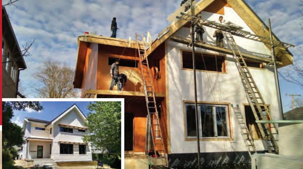
When Cedar Street Builders teamed up with Delv Design to produce Indiana's first passive house, the builders planned to achieve the required R-52 walls using SIPs construction but were confronted with a few hurdles.
