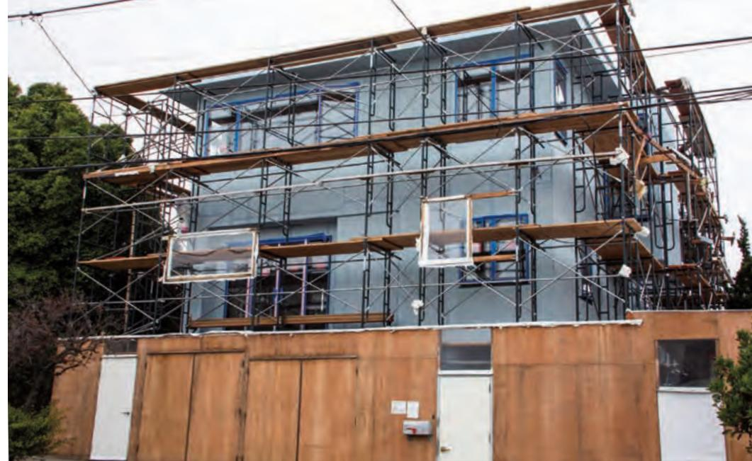
Solar panels will cover the roof, exceeding the anticipated energy loads to provide power back to the grid. The roof assembly consists of TGI framing, with an overlay of rigid insulation that tapers down from 6 inches at its greatest depth to 1 inch.
