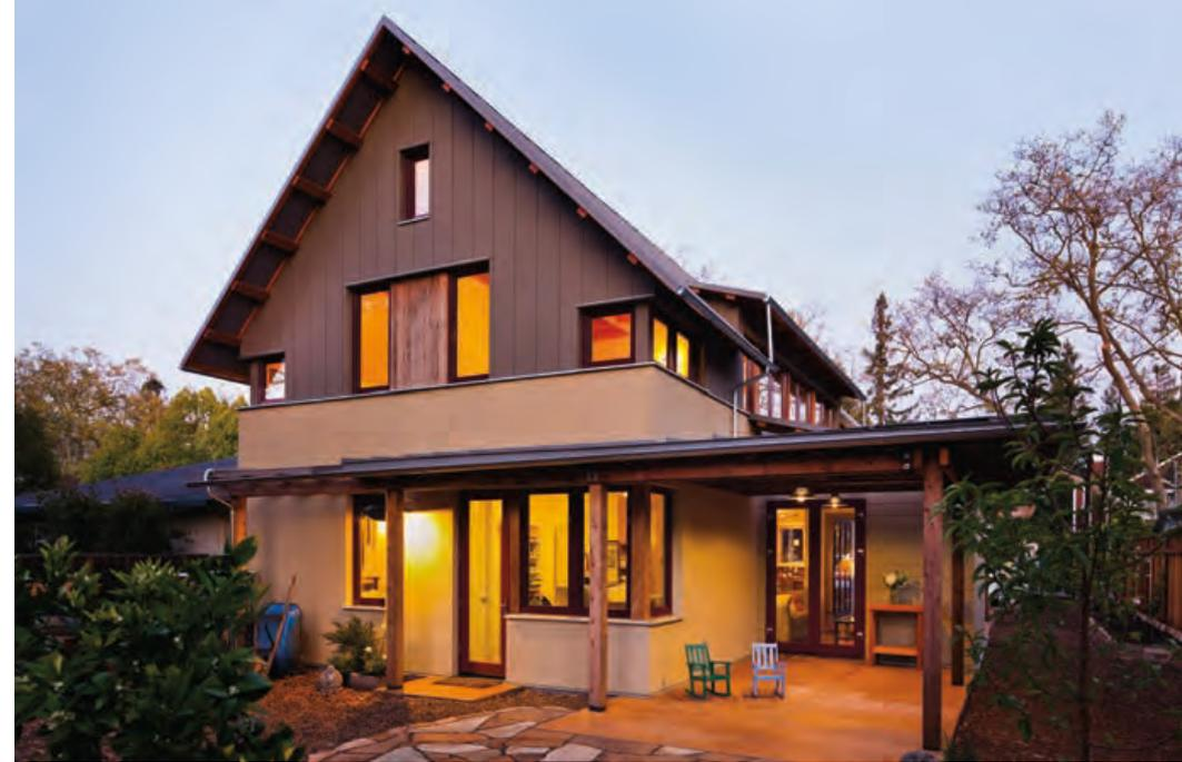
To minimize the use of non-renewable fuels such as natural gas, this house features an air-to-water heat pump that feeds a hydronic heating system, as well as an induction range—replacing the two most common consumers of natural gas in California homes with electric appliances. A PV system generates enough electricity to power these appliances and meet all of the family's other electricity needs on an annual basis.
