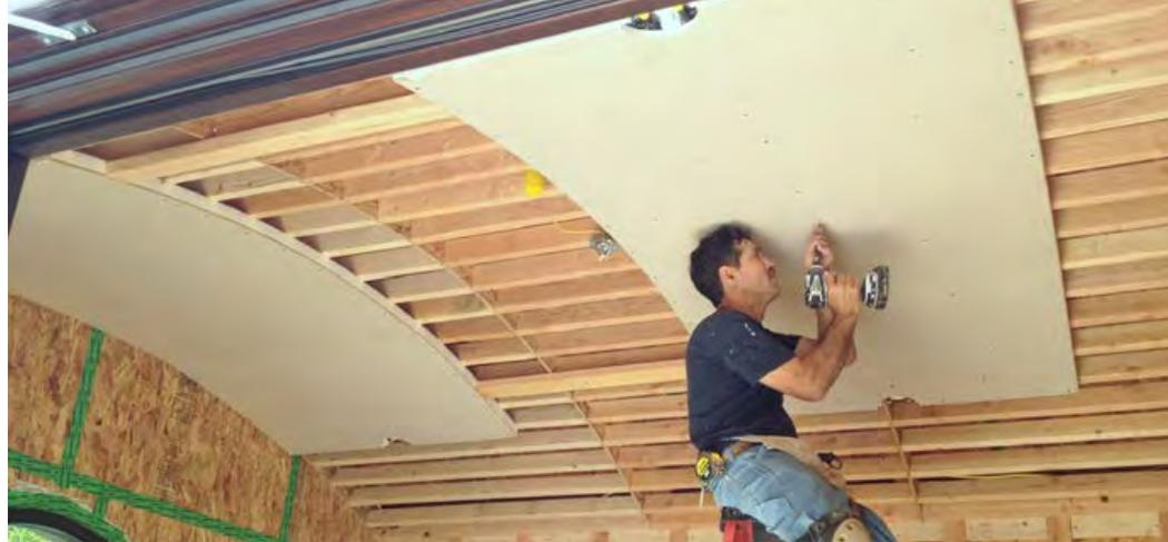
Spanish Colonial Passive House, Paolo Alto CA. Installation of Ray Magic radiant gypsum panels on a rounded ceiling. The piping layout is laser engraved on the paper surface of the panel for easy installation without puncturing pipes.
