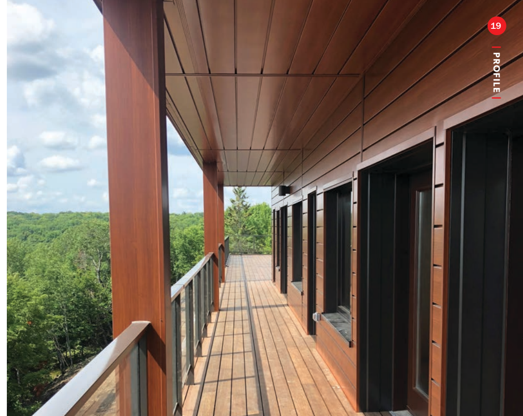
Photos by Greg West, Gwest Building Services
