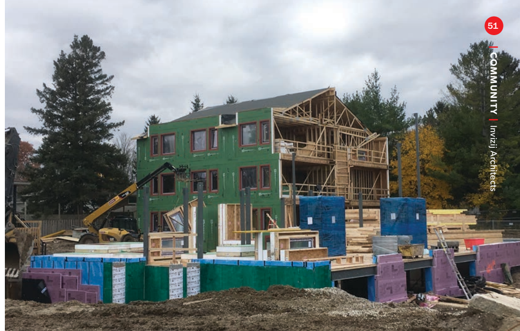
Photos by Greg Leskien, Zon Engineering
