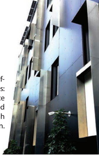
"The Battery" by Onion Flats in Philadelphia. Onion Flats will be using 28 PentaCare V12 units in its upcoming "Bank Flats" project this fall.
