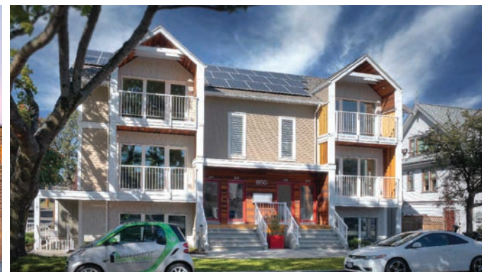
Alta Lake Passive House (top), BC Passive House Ltd. Factory (bottom left), and North Park Passive House (bottom right).
