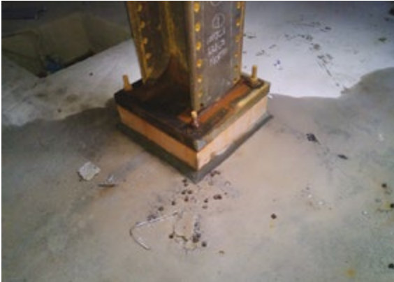
The beige color in the column base is 6-inch thick structural thermal break foam. This product’s compressive strength is higher than the concrete it sits on.
