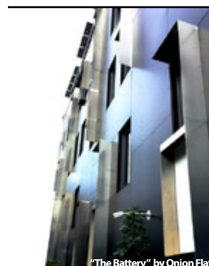
"The Battery" by Onion Flats Onion Flats is installing 28 PentaCare V12 in its actual "Front Flats" project in Philadelphia Q1-2019
